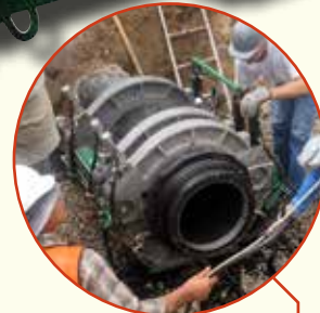
Quick 3- or 4-jaw conversion to allow unit to fit in tighter spaces
